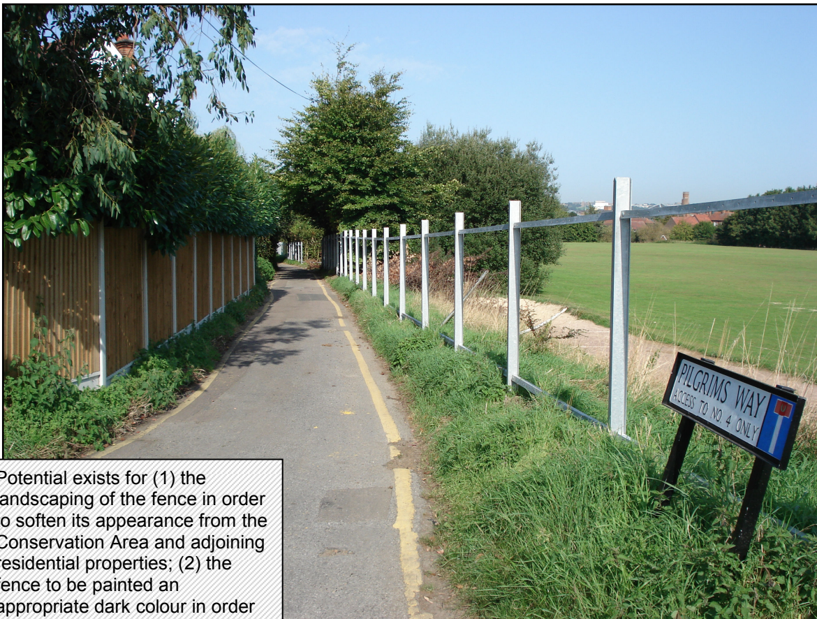
Figure 2 (below) – View of 1.8m high palisade fence currently installed along Pilgrims Way Public Right of Way
