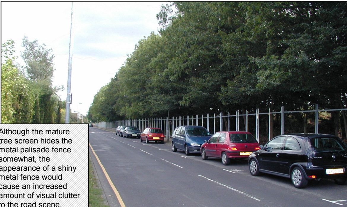
Figure 2 (below) – View of 1.8m high palisade fence currently installed along Pilgrims Way Public Right of Way
